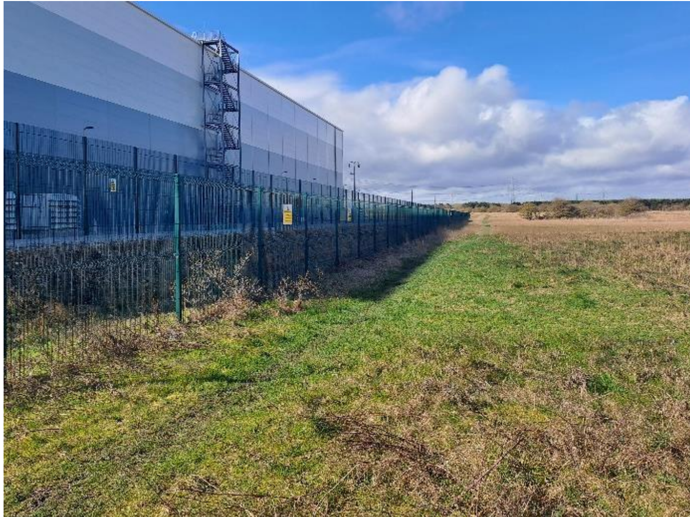
Figure 2.4: NSL Substation, near HVAC route (HVAC Zone)
