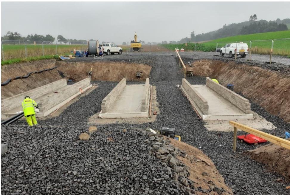
Plate 5-8 Example photograph of the construction of a joint bay
