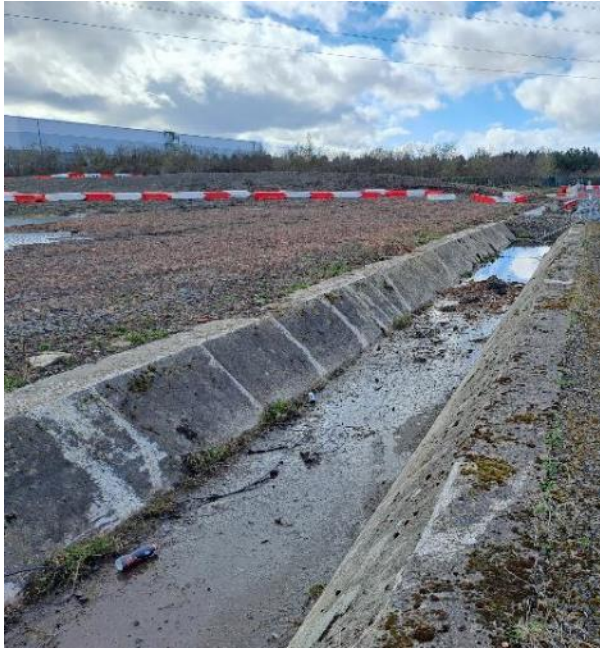
Photo 1: British Volt Site – Drainage and Hardstanding
