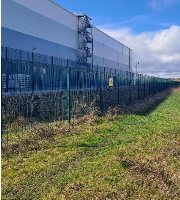
Photo 13: NorthSea Link Station
