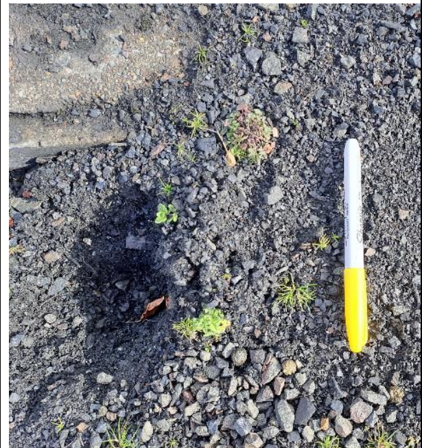
Photo 18: Colliery Spoil Type Material on Embankment
