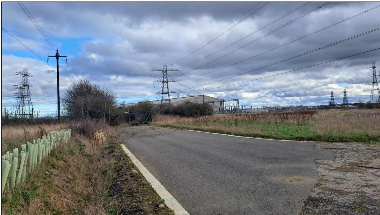
Photograph 13: (NZ 29637 83341) view southeast, toward the industrial site for which the roads are laid for
