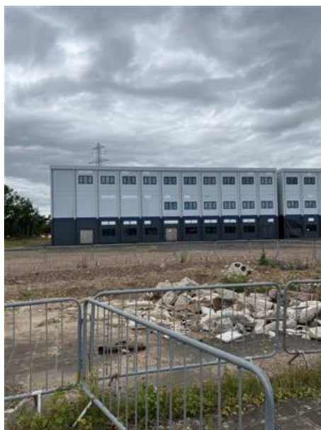
Photo 40: Single building on the former Britishvolt site
