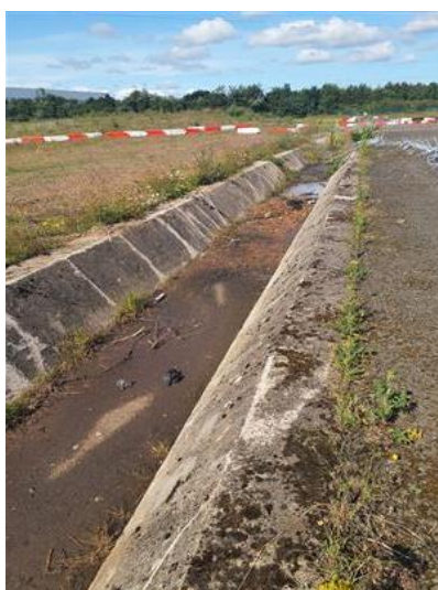
Photo 31: Examples of concrete based ditch
